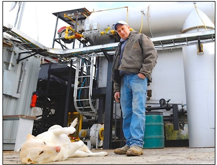
Figure 6: Josh Frye and his Gasifier
